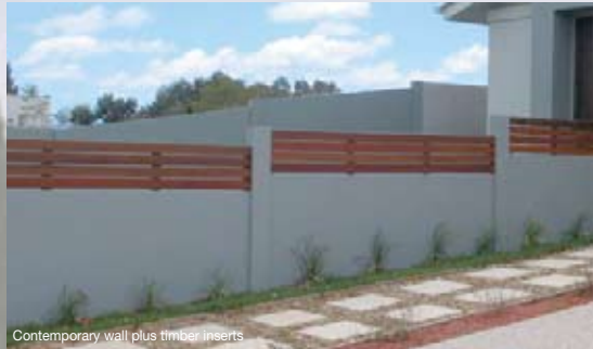
Contemporary wall plus timber inserts
